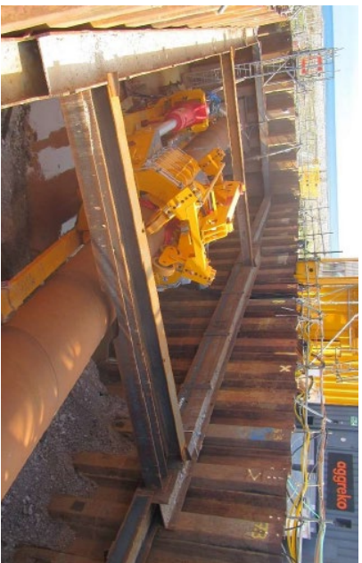
Plate 3.4: Direct pipe thruster equipment at the landfall compound
