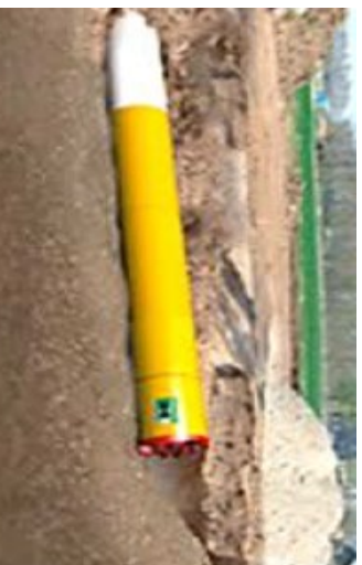
Plate 3.5: MTMB machine at exit location
