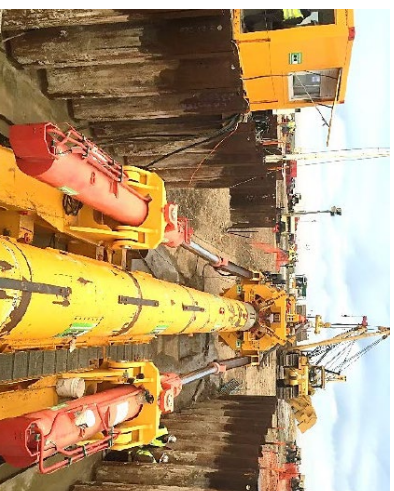
Plate 3.4: Direct pipe thruster equipment at the landfall compound
